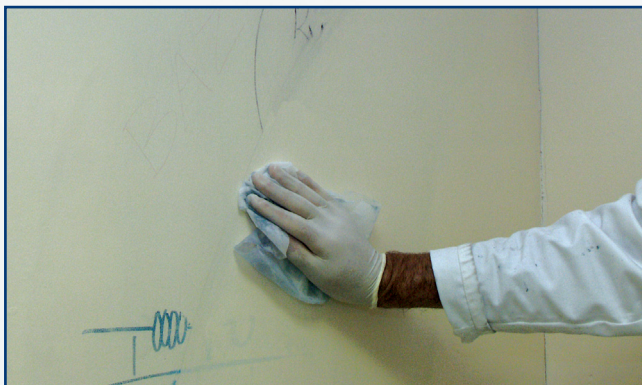
Graffiti removal in progress
